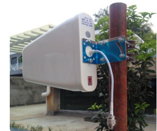
Step 2: Connect the outdoor antenna to the signal repeater BTS Port by cable. The joint of outdoor antenna and cable should be wrapped well with waterproof tape.
