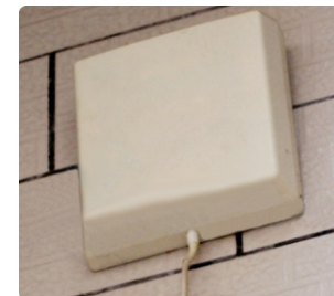
Step 3: Signal repeater MS Port connect to indoor antennas (Ceiling mount antenna or Panel antenna) by cable or directly connect to indoor antenna. If more than one antenna, please connect with the splitter first.
